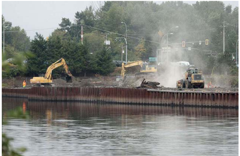
Figure 1: Heavy equipment working at Kus Kus Sum
