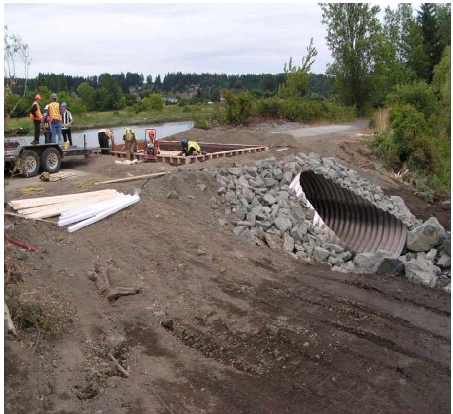
Figure 12: Project Watershed's Lagoon breach project
