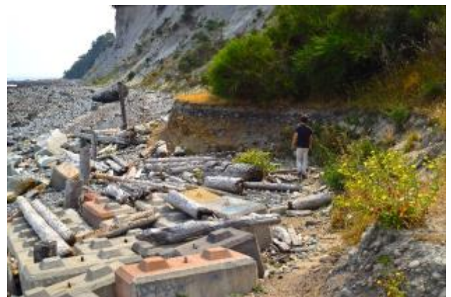
Modification of shoreline and erosion of attempted shoring at Cape Lazo, 2017.
