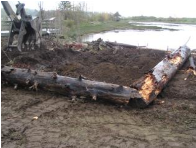
Excavation work at Courtenay Airpark.
