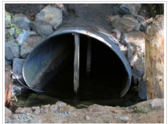
Culvert after water level is raised. Photo: K. Clouston
